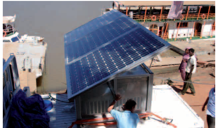
TWS 200: treatment of organically contaminated river water (Nile) in Khartoum, Sudan 2009
